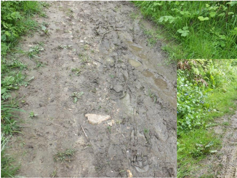
Typical rough and muddy surface condition elsewhere along BP1662
