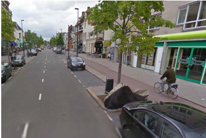
Example of cycle track passing behind parked cars (Biltstraat, Utrecht) 8
