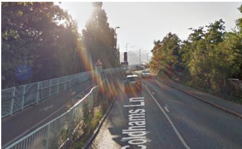
Coldhams Lane railway bridge, Cambridge
