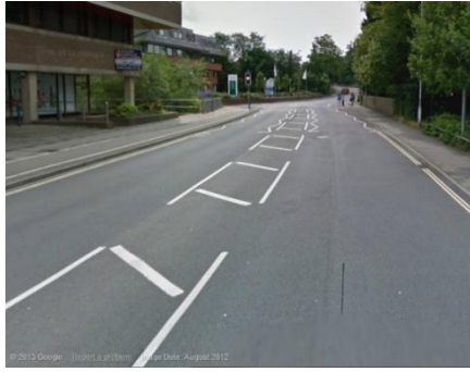
Central hatching in Worthing Rd reduces space for cyclists
