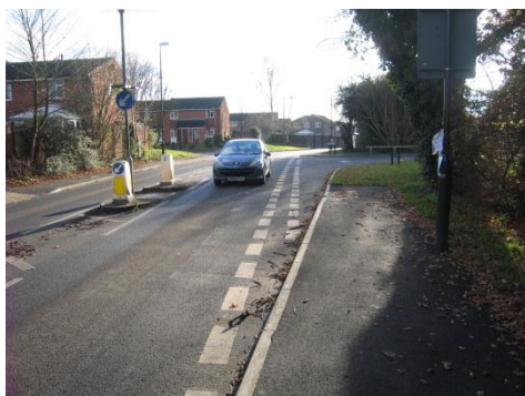
Excessive splay on new access road to Highwood
