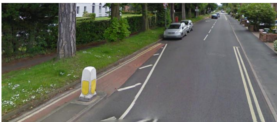
Cars parked at the end of poorly designed 'cycle facility' in Crawley Rd cause cyclists to swerve out into oncoming traffic
