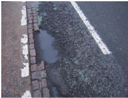
North Parade: main carriageway has been resurfaced twice. Chippings erode the cycle lane which has not been resurfaced at all.
